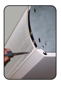
When making electrical connections first remove the safety cover plates over the electrical supply terminals. On 2m electric air curtains the safety cover plates are located towards the centre of the air curtain (See Insert).
